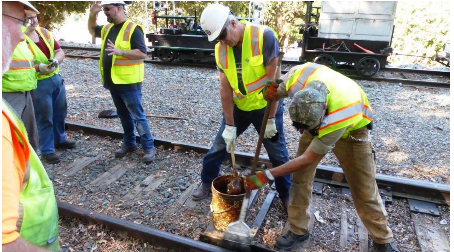
At Switch 15 (Setzer Lead) Kyle sweeps debris out from between the point and stock-rail as Scott goops up the grease brush with switch-grease
