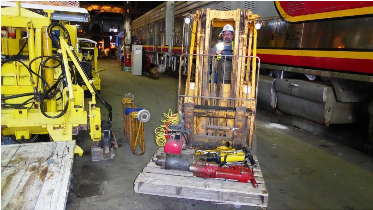
DJ brings the hydraulic tools over for loading on the flatcar
