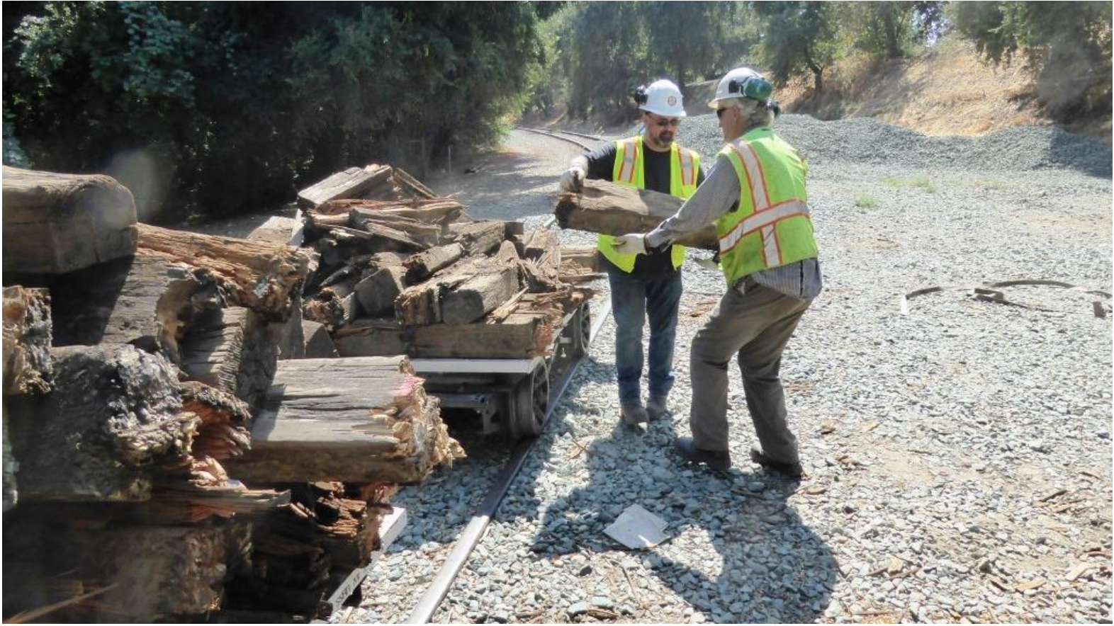
At Setzer, DJ and Steve unload the dead-tie debris...
