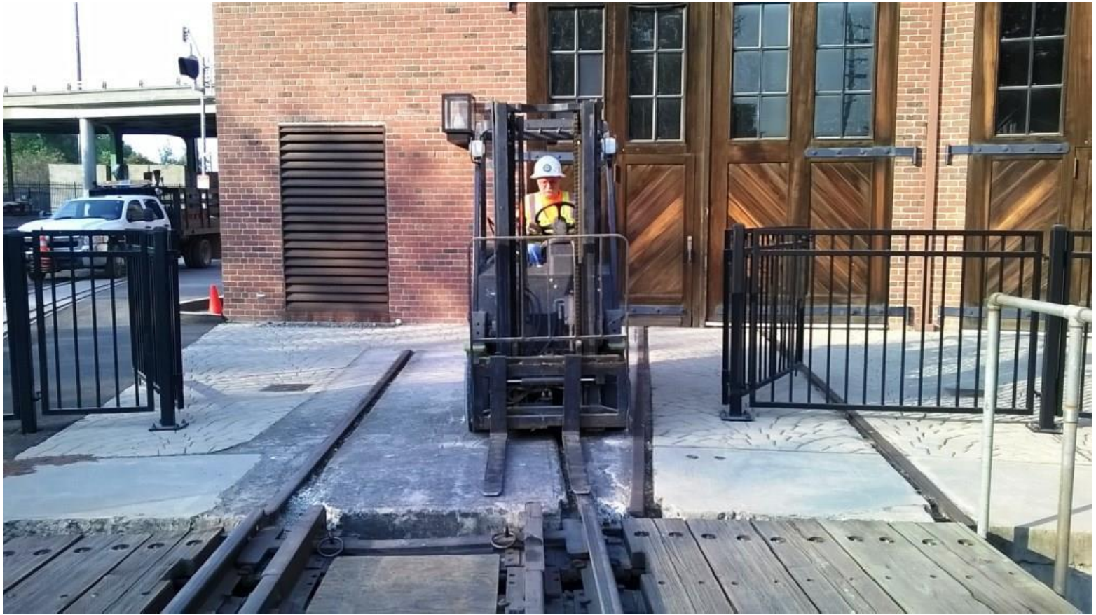
Mike H. uses the propane powered forklift to shimmy the wayward rail back into position
