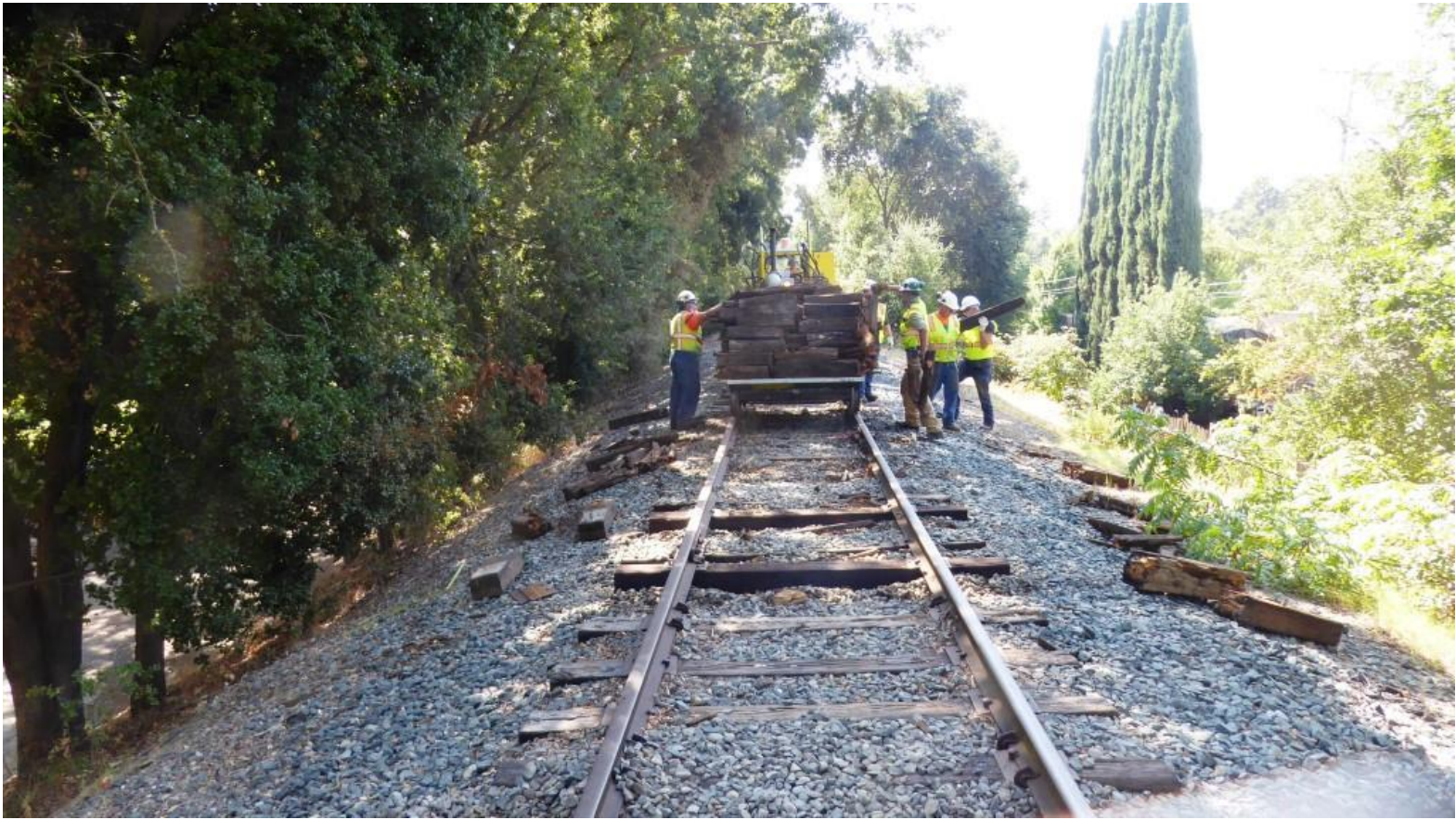
Meanwhile, Team Tie-debris loads the flats to capacity
