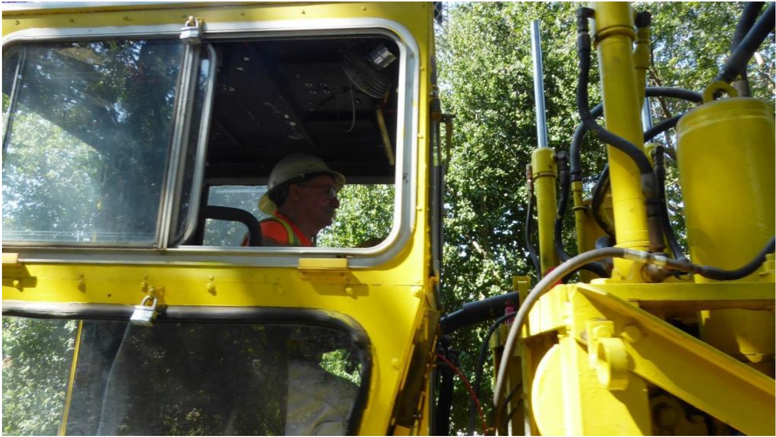
Mike H. at the controls of the tie-shear slowly moves up the line as the Team loads dead-tie debris on flatcars
