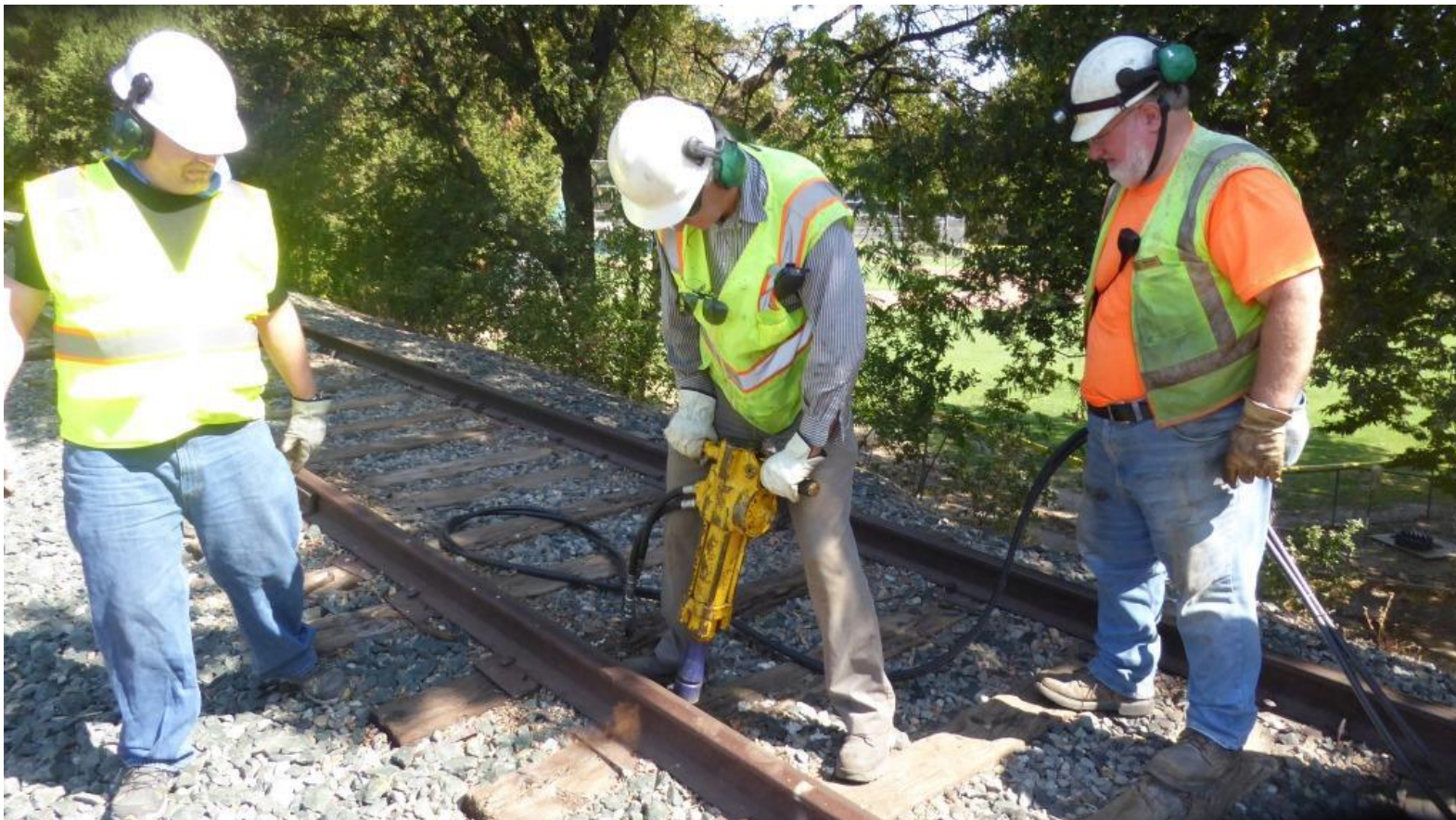
Although very disappointed that he couldn't drive spikes by hand with a spike-maul, Steve gives in and takes the hydraulic spike driver in hand as Frank minds the hydraulic hose
