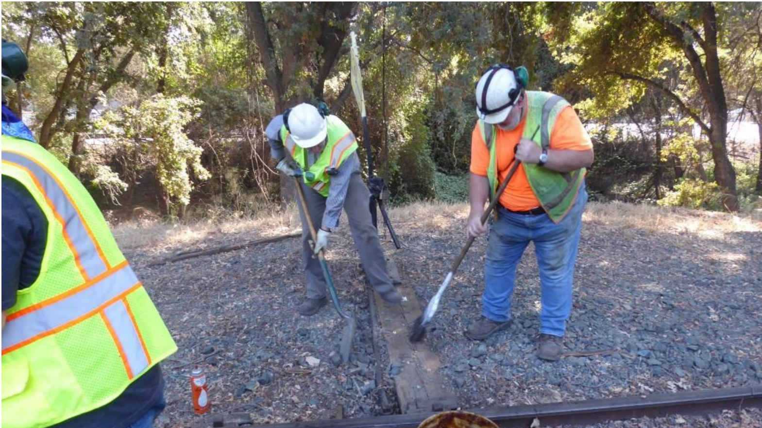
Steve and Frank clear obstructions from around the switch-rod and head-block
